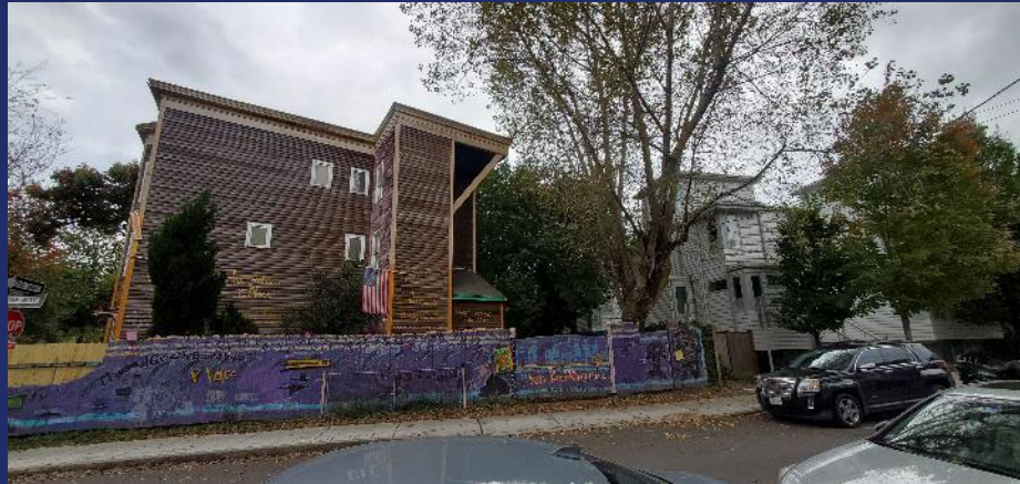
View from Franklin St.
