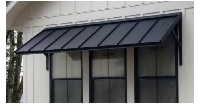
CANOPY STANDING SEAM METAL AWNING
