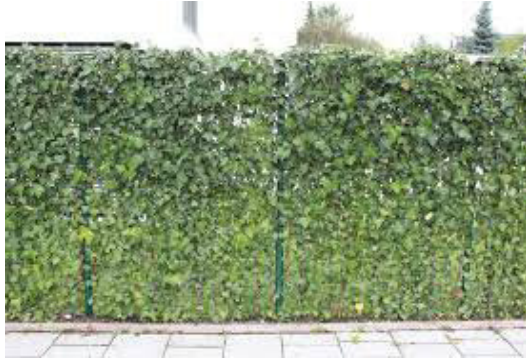
TRANSFORMER FENCE WITH IVY APPROX. 9' - 6" HIGH
